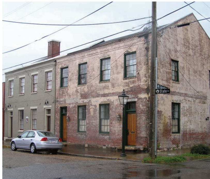
The home of Devereaux Bemis, Director of the Mobile Historic Development Commission was built in 1839 by the Batre family of Mobile. It was the site of the Model Grocery Store from 1916 until the mid-1990s.
