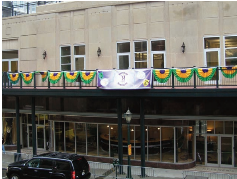
Hargrove and Associates, with a workforce of over 200, has renovated the Neisner Building and is working to bring life to the long shuttered Kress Building.
